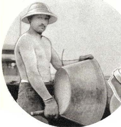
Chained over shaved pole butts, rubber tubs (above) hold termite-killing "medicine" which is supplied, under pressure, until chemicals have had ample time to impregnate the sap wood. Below—Placing a tub on butt.
