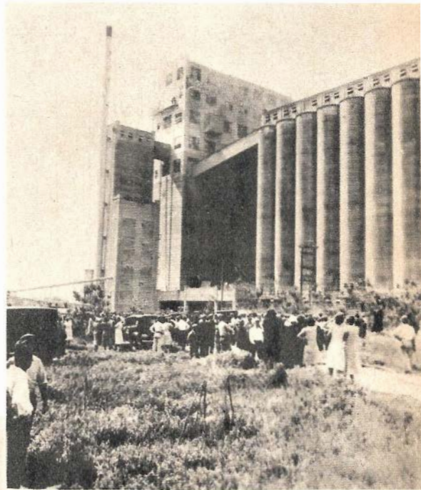
Six men were killed and six injured when a grain elevator in South St. Louis, Mo. (above), said to be one of the largest in the world, was added to the list of dust-blasted buildings. Relatives and friends await removal of victims' bodies by firemen. Note blown-out windows.
