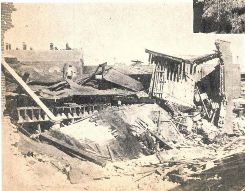
Six men were killed and six injured when a grain elevator in South St. Louis, Mo. (above), said to be one of the largest in the world, was added to the list of dust-blasted buildings. Relatives and friends await removal of victims' bodies by firemen. Note blown-out windows.
