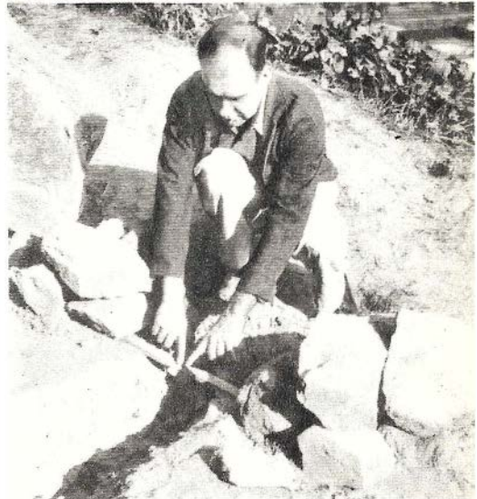
Top—Aerial view showing the mountain slide which menaces the homes of residents in a section of Los Angeles, Calif. Lower—Pointed sticks held over a crack on mountain's crest serve as a means of determining whether a new slide threatens.
