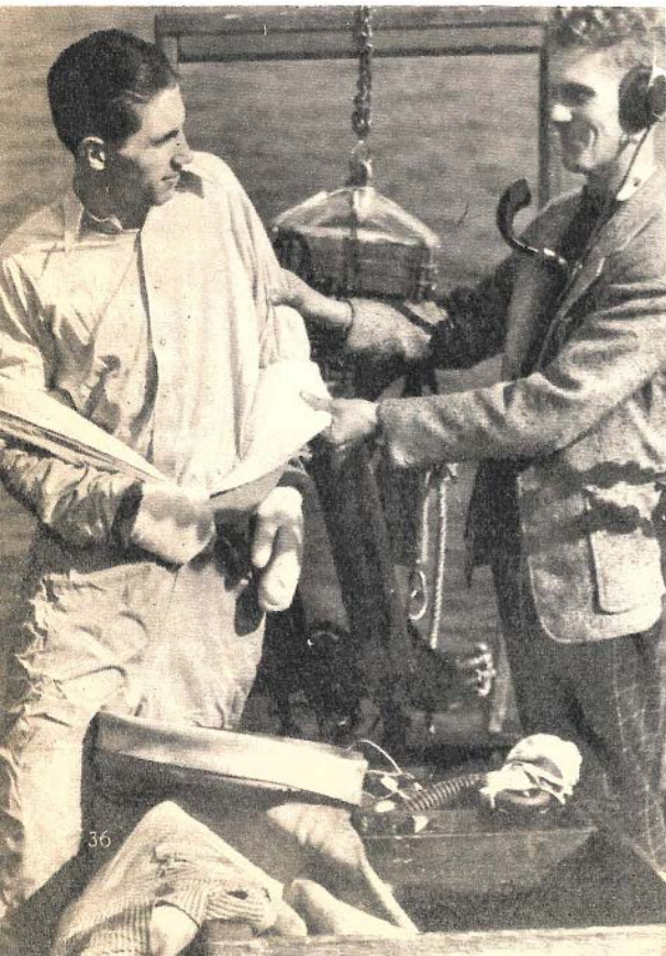
Diver Max Nohl, first human to breath helium under water, wears a fleece-lined canvas suit under the outer rubber suit, which is one-half-inch thick.
