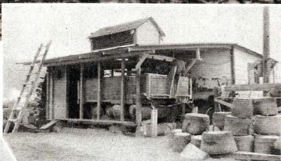
Above—The chemical mixing and storing plant. Below—This compressor provides constant pressure on chemicals in the rubber tubs clamped tightly around pole butts.
