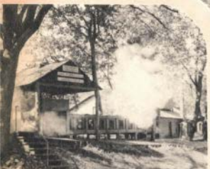
When dust from a million bushels of grain exploded in an elevator at Quincy, Ill., all that was left was the smoldering ruins shown above. Left—A U. S. Department of Agriculture testing station for conducting experiments with self-opening windows to determine their value in preventing damage from dust explosions by releasing explosion's pressure. Note explosive flames leaving window.
