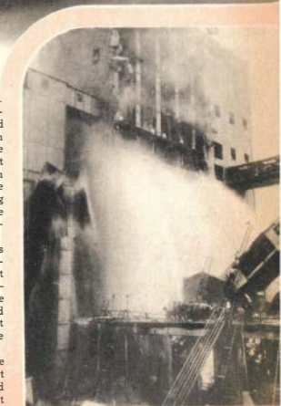
Five successive explosions of combustible dust virtually blew the entire wall out of a twelve-story grain elevator in Baltimore, Maryland, as shown above.
