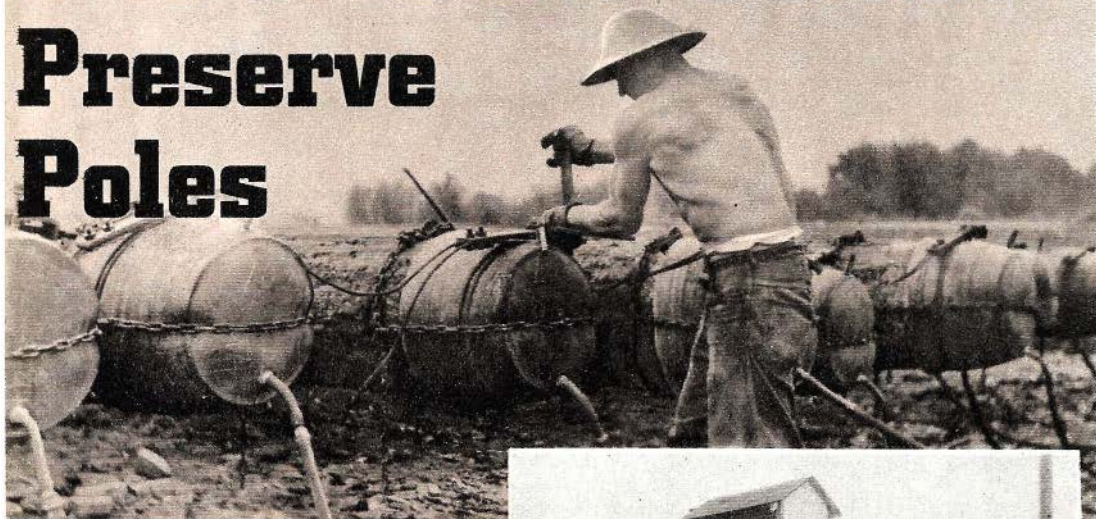
Chained over shaved pole butts, rubber tubs (above) hold termite-killing "medicine" which is supplied, under pressure, until chemicals have had ample time to impregnate the sap wood. Below—Placing a tub on butt.
