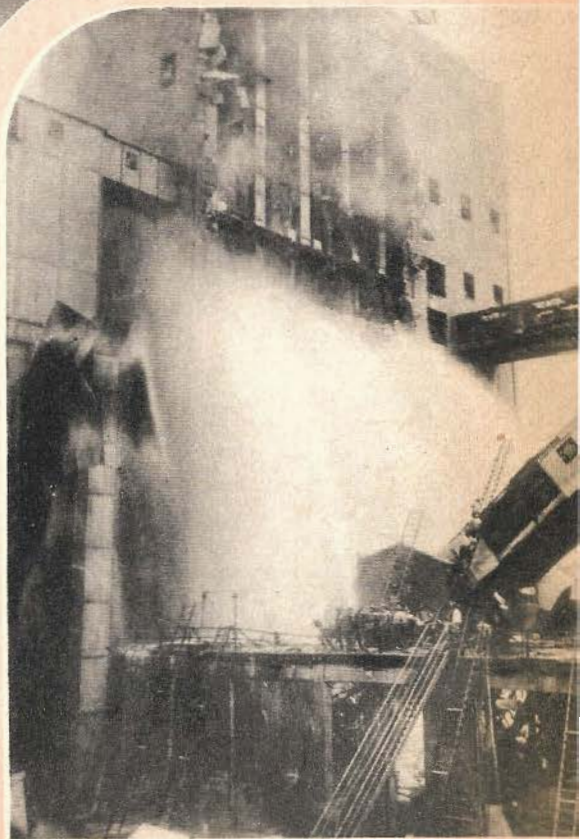
Five successive explosions of combustible dust virtually tore the entire wall out of a twelve-story grain elevator in Baltimore, Maryland, as shown above.
